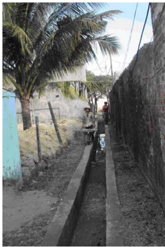
Figure 21. Executing drainage in Sections 29, 30
