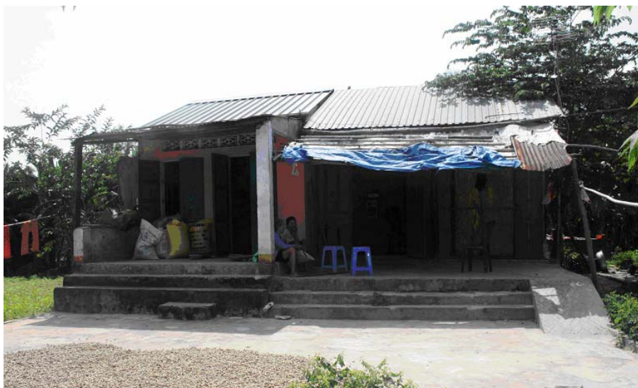
Figure 24. For convenience, Mrs Boi (Sect 37) still uses temporary house next to a brick house.
