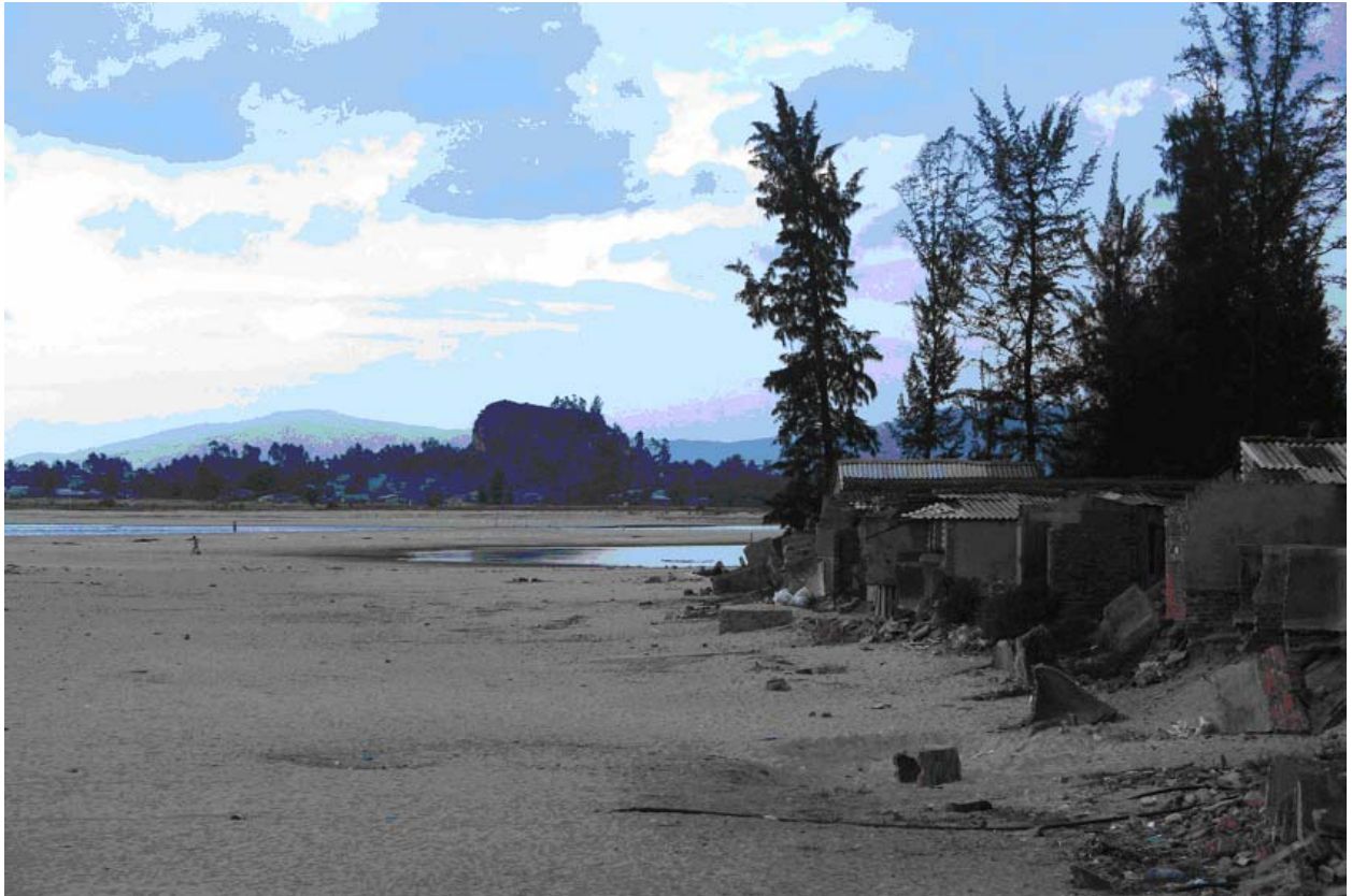
Figure 17. Shoreline erosion damaged houses and tiger shrimp hatchery station, Hoa Hiep Bac
