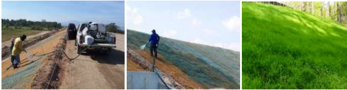
SLOPE SOIL STABILIZATION THROUGH HYDROSEEDING TECHNIQUES
